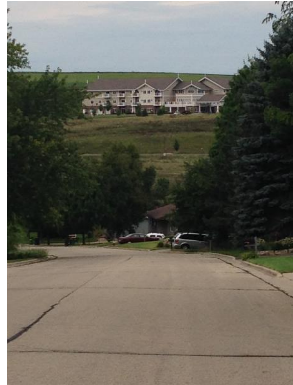
New Glarus's steep roads can create maintenance and stormwater management challenges.
